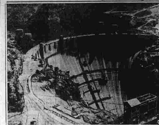
nt. The creet of the dam is strikingly shown above, with the roadway is the open to the public. This will afford a good route from Las Vegas, he tower tops can be seen over the dam and the Arisona spillway, is at the extreme right.
